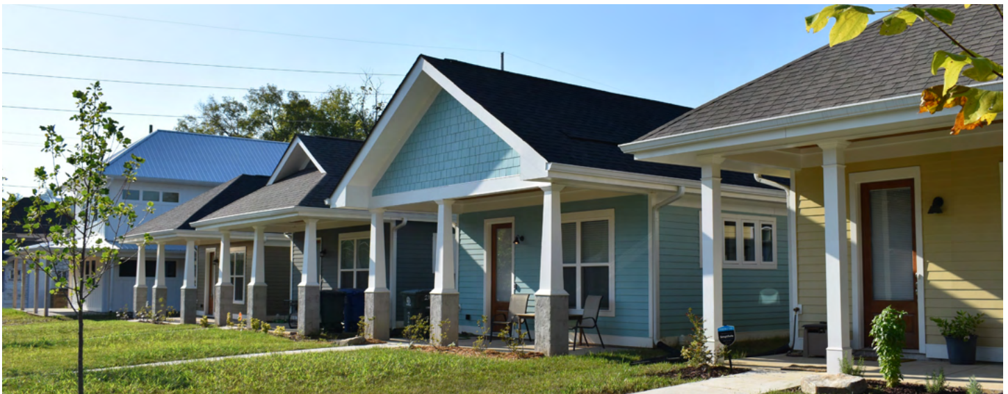
Finished row of cottages on Union Ave
