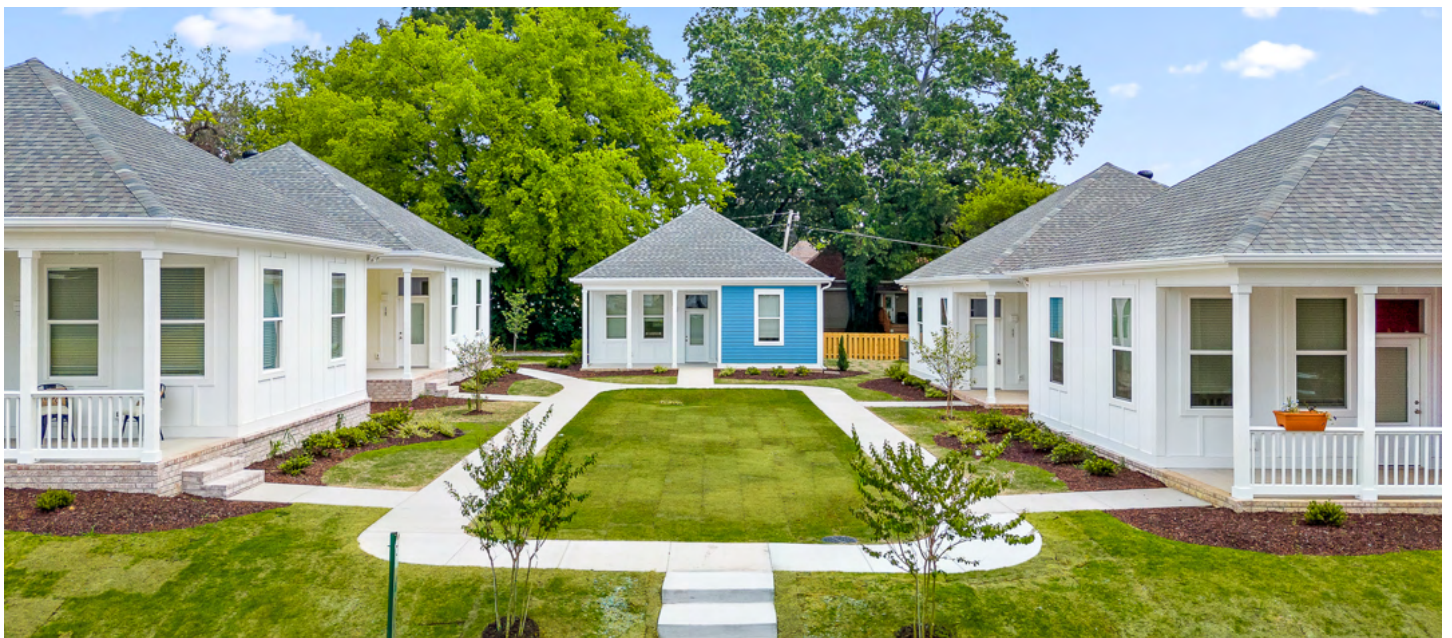
Finished Cottage Court on Vance Ave
